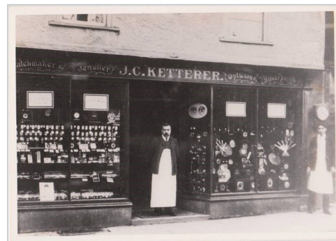
It is possible Ketterer occupied the same premises as Mary Ann. This photograph was taken circa 1910. This is the same shop as J E Allnut & Son now occupy
